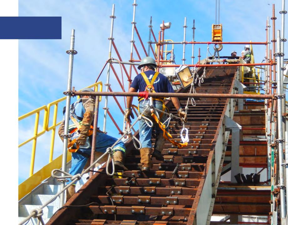
These extensions, combined with elevating the chain return rail, increased the area required to meet the capacity without increasing chain speed.
